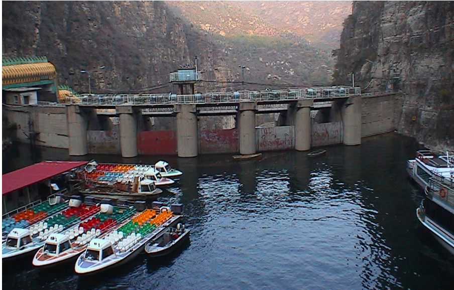
Fig. 1. The reservoir of a mountain hydro-power plant (China)
