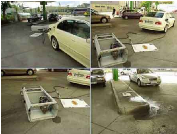
Fig.1. The accident that occurred due to not pulled out of a tank a filling pistol
